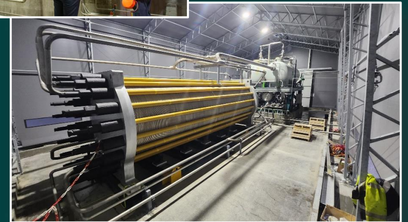
HQ and test center at Herøya, Porsgrunn
