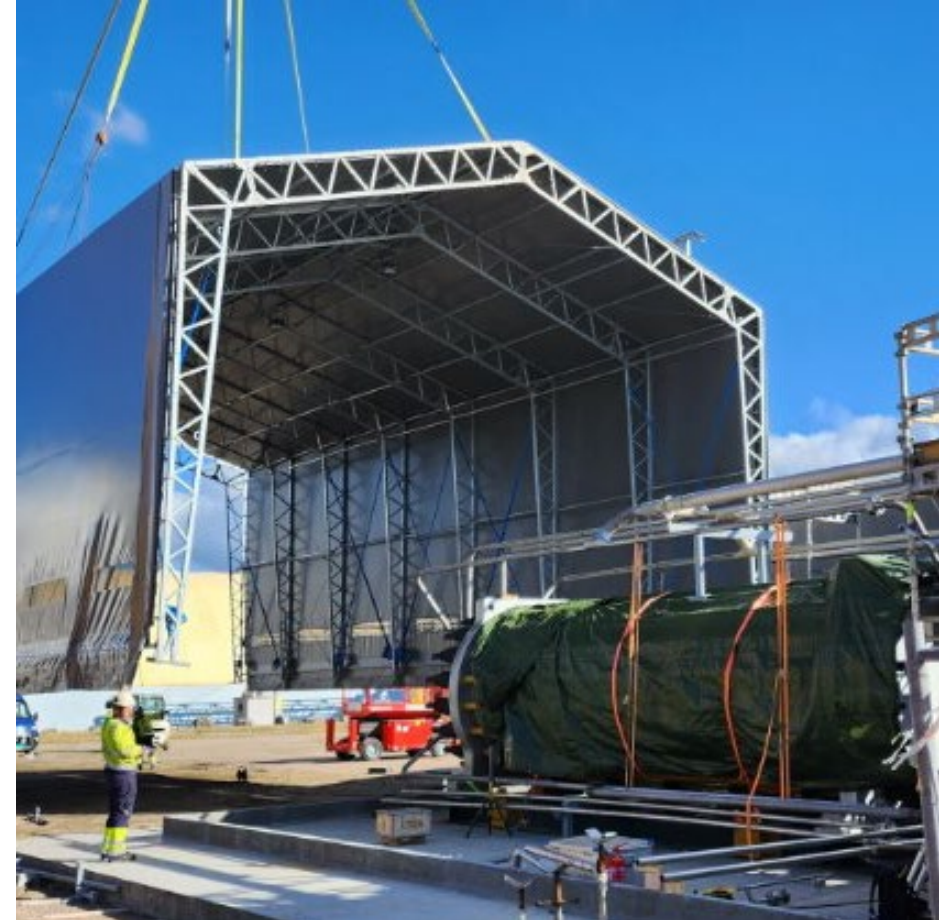
Installation of HydrogenPro's facility at Herøya, Norway in September 2022
